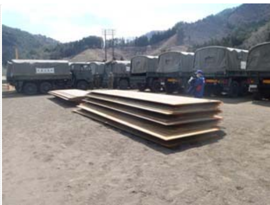
敷鉄板数量確認 (4/3)
