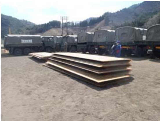
敷鉄板数量確認 (4/3)
